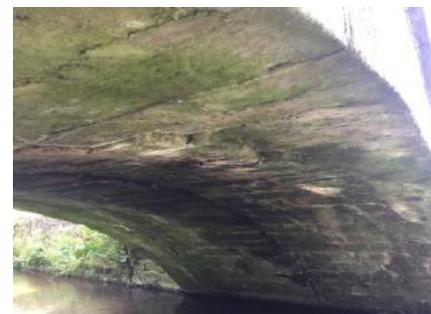
the first operation was the design and install of a temporary works propping system to hold the arch in place allowing access above with plant and equipment and to allow the fallen stones to be jacked back into position.
