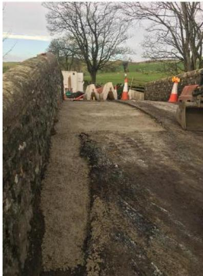
Once installed the surfacing from the structure could be removed exposing the bridge arch, this then allowed the engineering team to monitor accurately the jacking of the bridge structure back to its correct alignment.
