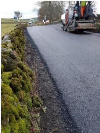
The works had to be undertaken under a full road closure due to the width of the road and 3 x Tie-ins cold milled to accept 100mm AC 32 HDM 40/60 Base Course, 50mm of AC 20 HDM 40/60 and 50mm of HRA 30/14 PMB WTR2 and 60 PSV Pre Coated Chippings. Tanker applied bond coat were used for each layer before surfacing commenced.
