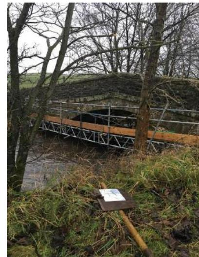
This involved core drilling through the entire structure, installing 40mm dia stainless steel tie rods then tensioning them and grouting them into position. To do this the Hinko scaffolding team installed a walkway across the watercourse allowing access for this operation.
