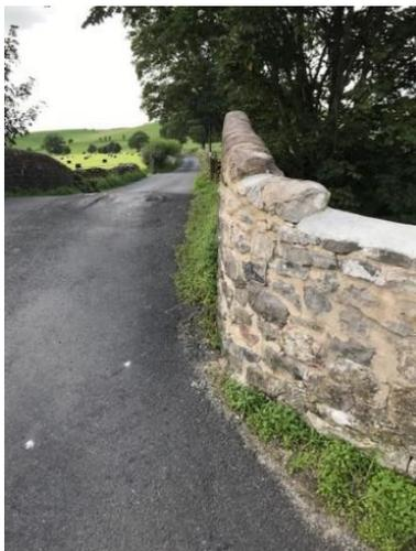
The process worked well and simultaneously work to the dam parapet could be undertaken by suitably qualified stone masons. As the structure is grade II listed, careful cataloguing of each stone was required to ensure that it was replaced in the correct position. Hinko's in house resource carried out these works.
