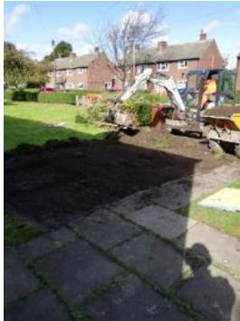
The original design showed gravel soak away's. The Hinko site management team proposed the use of Rain Bloc attenuation which was accepted by the Client and installed by the Hinko teams.
