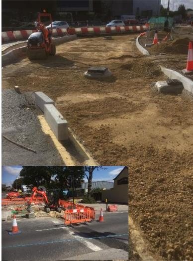
The initial works focused on stats diversions, junction realignments, new lighting infrastructure, kerb line and drainage / ducting install. This opened up areas up for the flagging teams to install the 8000m<sup>2</sup> of flags required.
