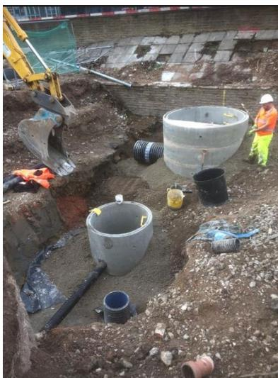
This system then tied onto new pipework and a series of pre-cast concrete culvert sections, eventually discharging through a hydro break into the waste water system.
