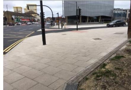
The works included full depth road construction where the carriageway needed widening to accommodate new bus lanes and turnings.
