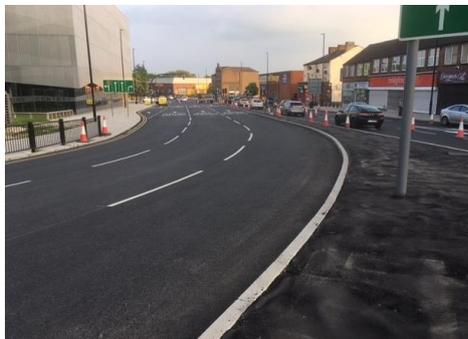
Once the kerb lines, road widenings and flagging works were complete the existing carriageway was profile planed and re-surfacing undertaken. These works were planned over a six-week period, split into manageable sections. To avoid major impact to pedestrians and road users, the Hinko team ensured that all the works were undertaken on night time road closures, this allowed the team to achieve their outputs and minimised disruption.
