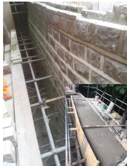
Once the concrete was fully installed then the new parapet wall could be re-built.
