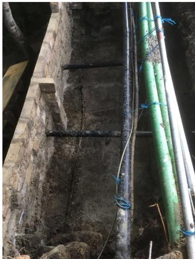
It was found that the sub-formation was primarily mud stone allowing for an almost vertical face to be cut out of the embankments without fear of collapse.
