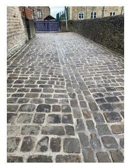
Once the setts were bedded into position, they were finished off by using a high flow grout making the sets and concrete bedding material below fully integral.
