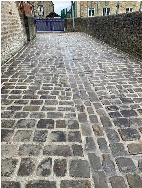
Once the sets were bedded into position, they were finished off by using a high flow grout making the sets and concrete bedding material below fully integral.
