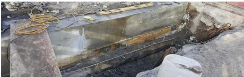
Once the diaphragm was complete the site team could then construct the new Ballast Wall, this was offset 30mm to allow for bridge movement.
