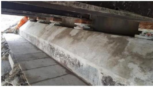
Simultaneously the site team worked on the bridges bearing shelves replacing the Honel Drains and bearings. Once complete the structure was released from the temporary works and the bridge rested on the new bearings.
