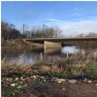
The structure has suffered from settlement and rotation at its abutments over the last 30 years to the point where the expansion gap at the structures free end was fully closed, thus the bridge was not moving as per its design.
