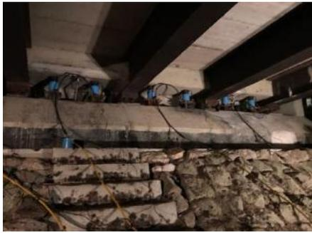
The structure was jacked to level on a night closure of the road, once to level temporary works packers were in place temporary ramps were installed to accommodate the new road level.
