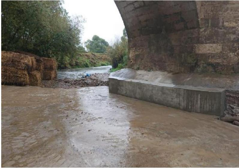
Throughout the duration of the project, inclement weather and heavy rainfall was a continuous issue. River levels would rise and breach the level of the temporary dam resulting in slowed outputs from operatives on the ground. This was continually monitored to ensure the safety of operatives was the first priority, all works were undertaken and completed during phase 1 of the invert protection slab.
