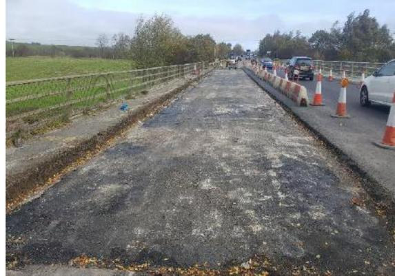
Concrete repairs were required at the location of the existing joint, these became evident post removal, shuttering was installed and subsequent repairs were undertaken using rapid setting mortar, this allowed minimal delays to stage one of the waterproofing system application.
