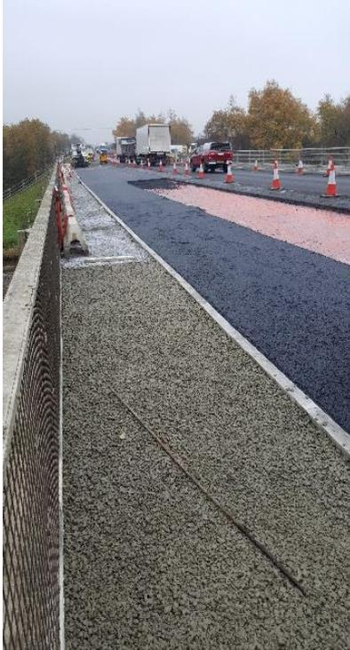
Once all contracted works on the North Side of the Bridge was completed, including cold milling, the second visit for the spray applied waterproofing works, Parapet mesh replacement, kerb installation and concrete verge infill, stage 2 of the surfacing was able to take place. This was to complete all binder course on the project. Surfacing was completed on time. Following on from this, Stage 3 of the surfacing was able to commence. Stage 3 would see
