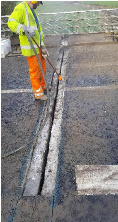
Over a single weekend, both nosing joints on the bridge were installed to the required specification. The joints were installed in 2 halves, 2No gangs working on each end of the bridge concurrently. When the first half was completed, a TM switch was implemented and the process repeated until both joints were fully installed.
