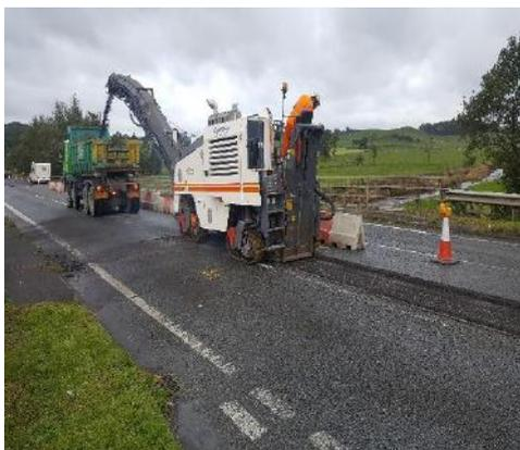
The initial works focused on traffic management establishment and cold milling of the existing surfacing to expose the bridge deck for preparation works for new waterproofing.
