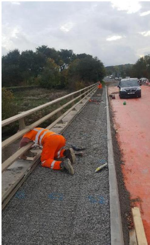
Parapet mesh was removed and replaced prior to stage 1 surfacing works. This was to ensure minimal disruption to the surfacing operations. The contracted stated any defective areas of grout on the parapet posts should be removed and replaced. This was completed in a timely manner prior to the replacement mesh being fitted.
