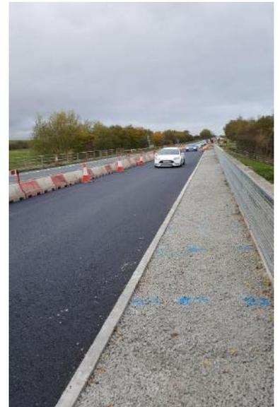
Bridge deck drainage was installed in 2 halves prior to surfacing taking place.
