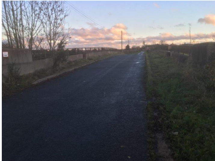
Eggbrough Lane Prior to commencement on site
