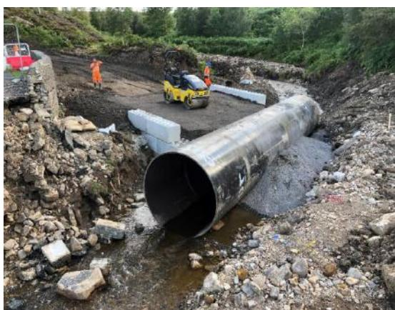
Hinko found that Pre-cast concrete culverts or pipes were not readily available, but the Hinko team quickly sourced large steel tubes from Cleveland Steel and Tubes, near Thirsk, had two disused parts of a Scottish wind turbine, which were cut to length, transported to the remote site and lowered into place so the road could be built over them.
