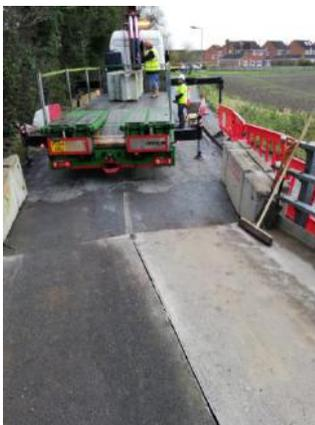
Once in position Concrete VTCB's were positioned at the four corners of the bridge on a splay to guide traffic in and also act as a retaining structure for ramps required either side of the bridge.
