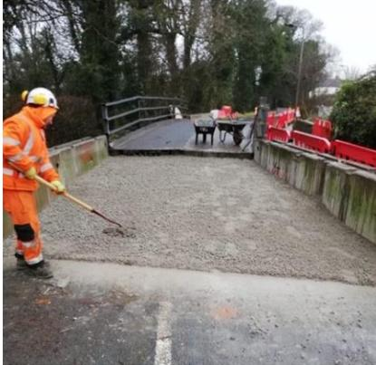
Once the TVCB's were positioned and utilising our in-house resource two No concrete ramps at a 1:12 gradient were constructed at each end of the bridge. This concrete was left 200mm down from Finished Road levels using our in-house resource
