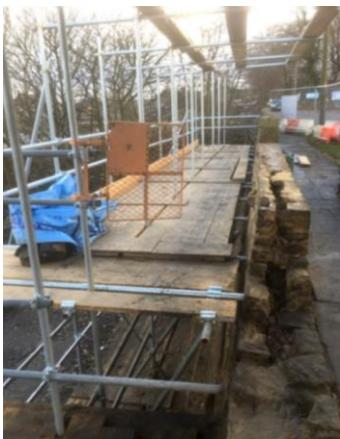
The works involved re-building sections of the existing wall, raking and pressure pointing the existing wall joints, and pressure grouting to the rear of the wall, and increasing the height of the existing parapet to a complaint level. This also includes temporary works and access.
