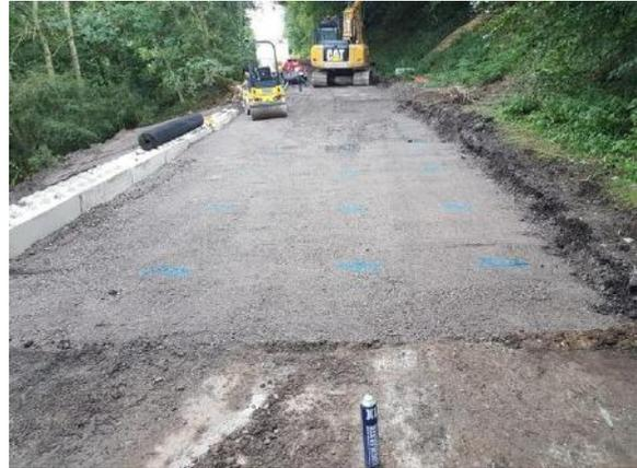
Once to level the road was capped off to formation level using Type 1 stone before the carriageway resurfacing operation was undertaken utilising Hinko's in house surfacing team.
