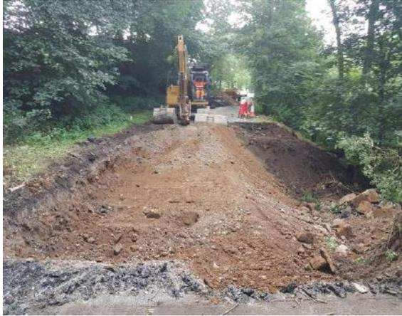
The first operation was to remove the remaining B6270 carriageway to enable a safe procedure to build up a permanent retaining wall. Hinko acted quickly, utilising its local supply chain to ensure that the procurement of materials did not delay the works.
