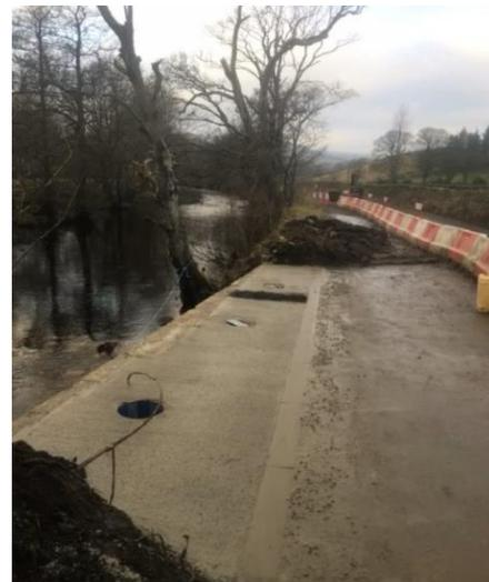
Once the wall was built to level rip rap was placed in the river to the front of the wall to protect the foundations from further scouring and also offered habitat for ecology.
